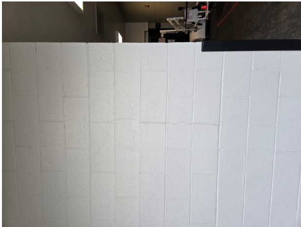
Vertical CMU crack (photo rotated).
