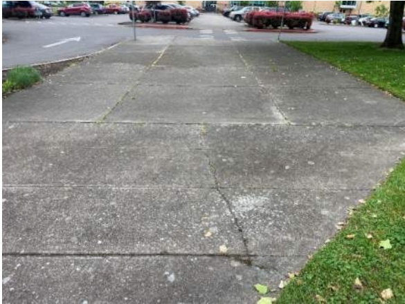
Photo 11: Longitudinal Crack in Route 3
