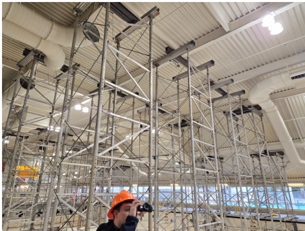
Existing natatorium roof shoring.
