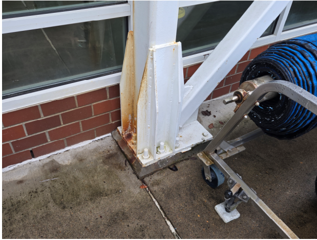
Surface rust at natatorium north wall braced frame column base.
