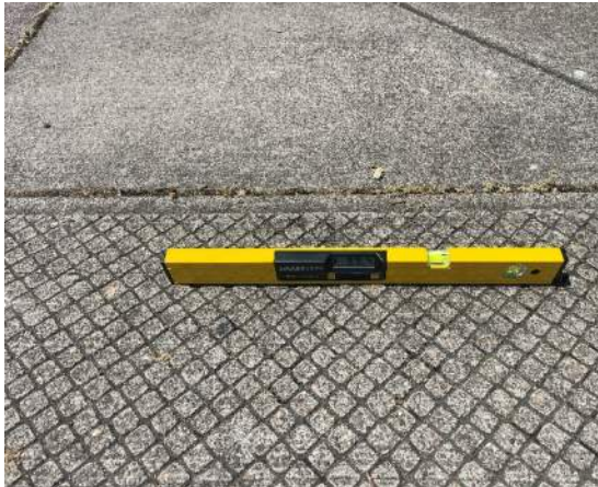
Photo 7: Route 2 East Ramp Run not compliant with ADA Standards (Ramp Run > 8.3%)
