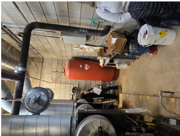
Unbraced tank in natatorium mechanical room (photo rotated).
