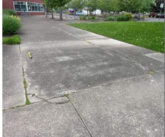
Photo 4: Longitudinal cracks and gaps present in Route 1
