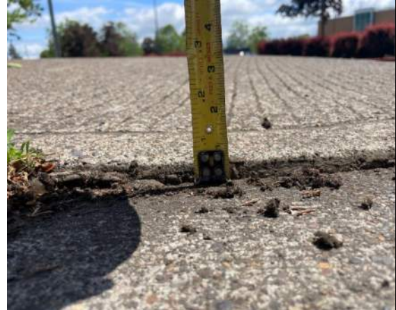
Photo 6: Route 2 East Ramp Run not compliant with ADA Standards (Lip > 0.25")
