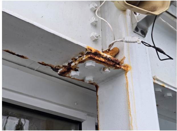
Natatorium north wall connection deterioration.
