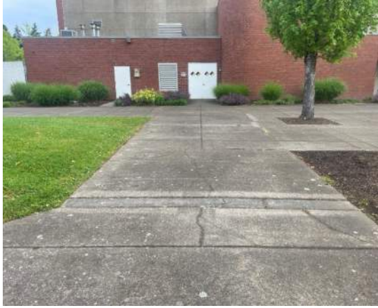
Photo 5: Longitudinal cracks and gaps present in Route 2
