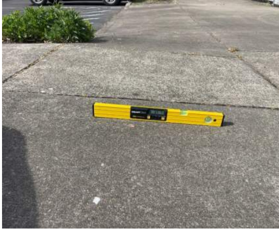
Photo 3: Route 1 East Ramp longitudinal approach not compliant with ADA Standards
