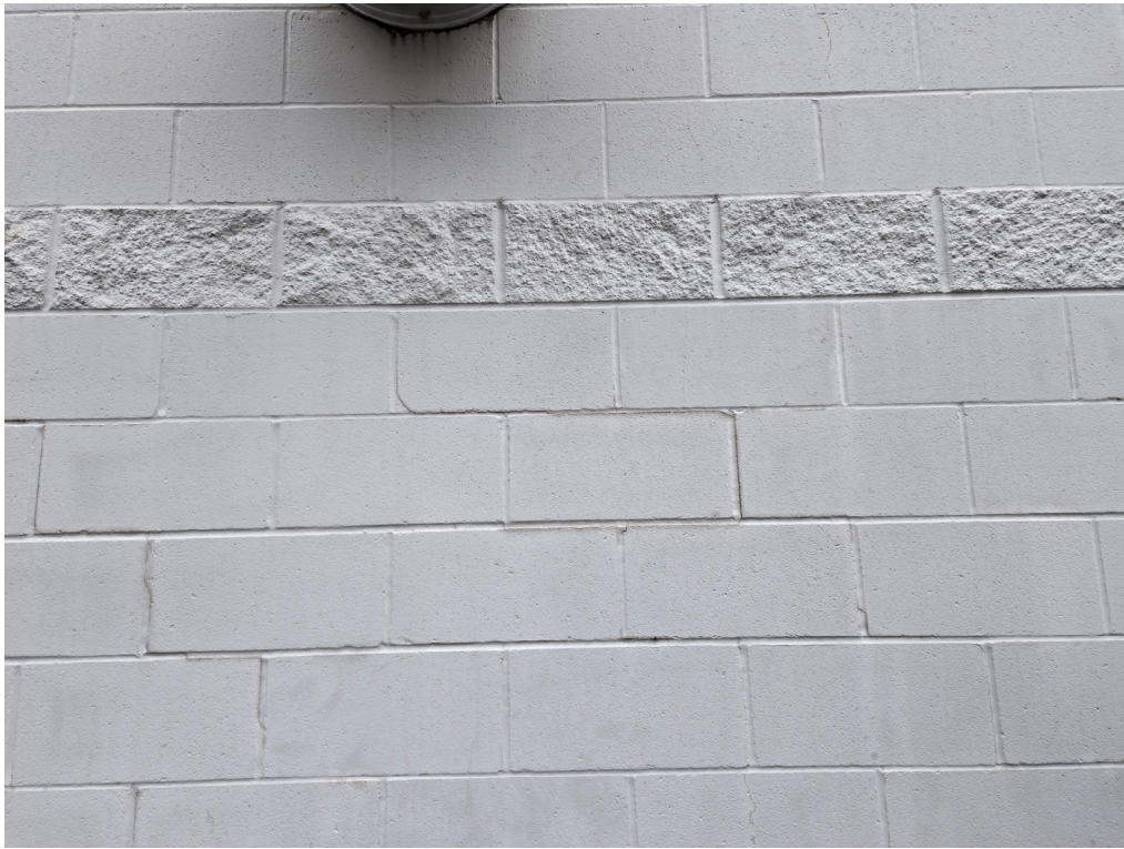
Examples of CMU cracking at detached pool building.
