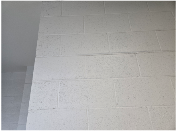
Horizontal crack in non-structural CMU wall.
