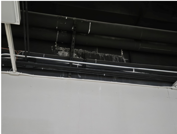
Evidence of interior moisture at natatorium south wall.
