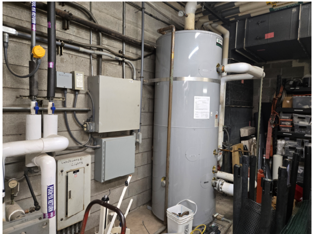
Partially braced tank.
