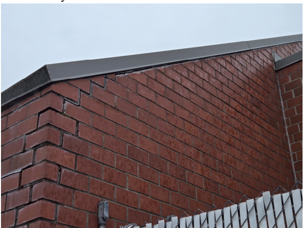
Northwest parapet veneer damage.
