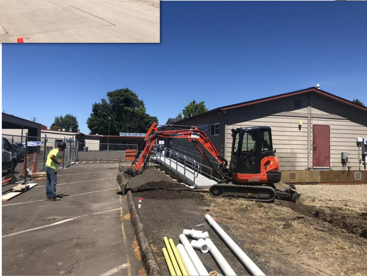
Lincoln – Viewmont work, clinic relocation and gym foundations
