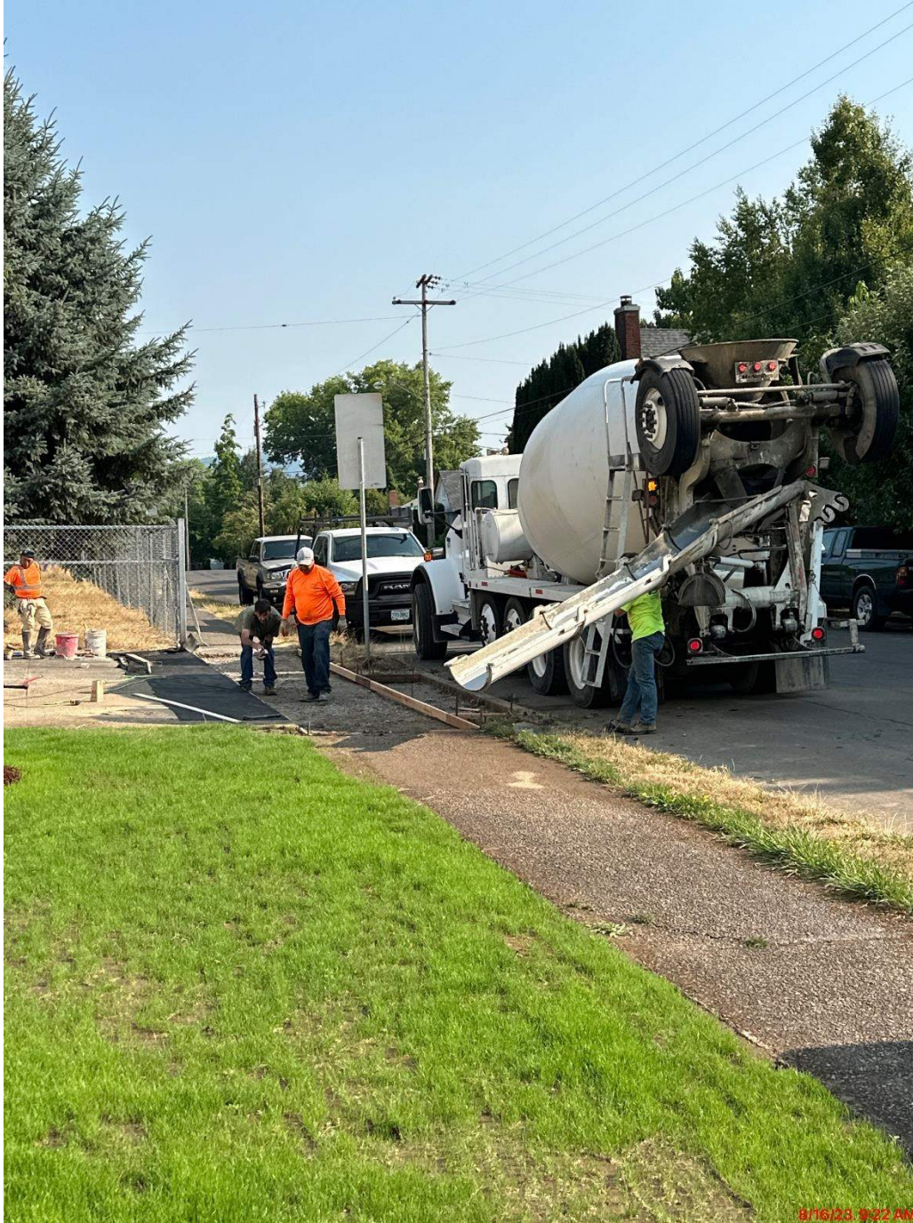
PIPC Repairs to Damaged Sidewalks
