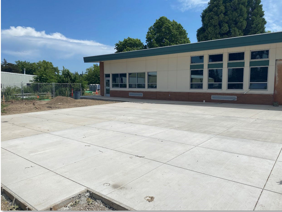
North Patio at New Addition
