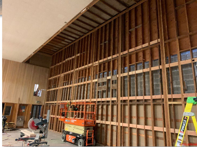
Gym Seismic Improvements
