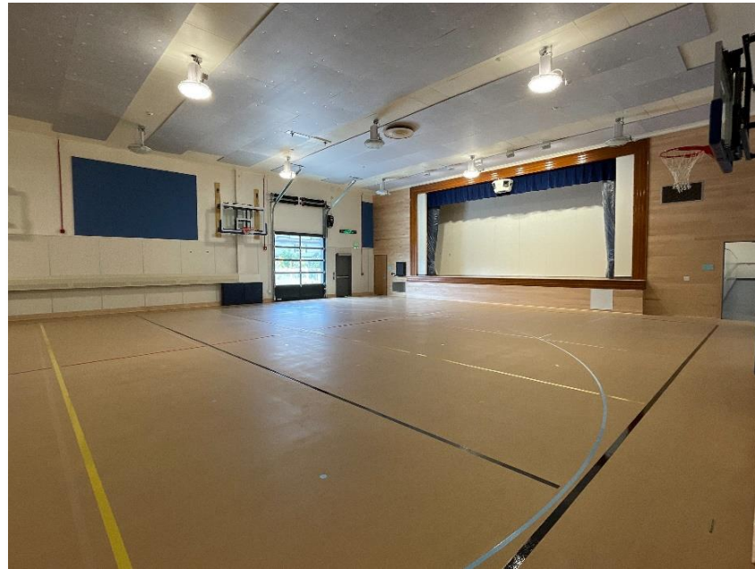
Renovated Gym Including Roll-Up Door to Outdoor Patio & Folding Partition to Library Space
