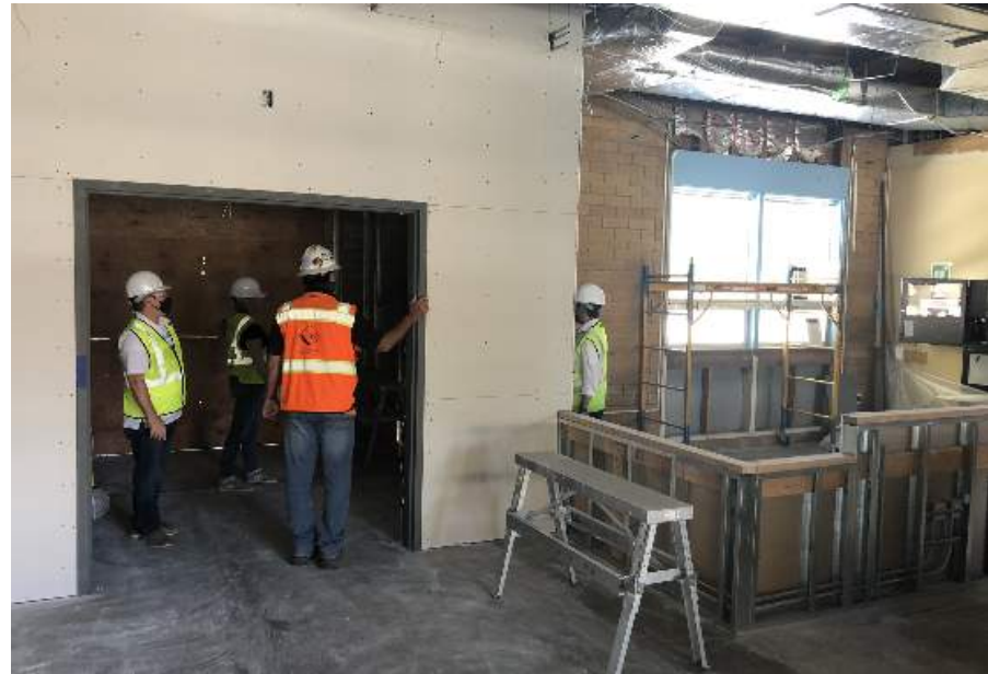
New secure entry vestibule and front office renovations
