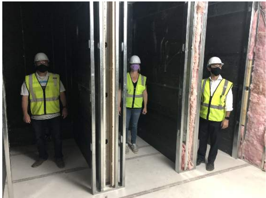
Inspecting the individual student restroom construction
