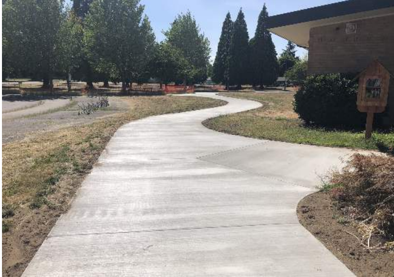
New ADA accessible sidewalk at front of school
