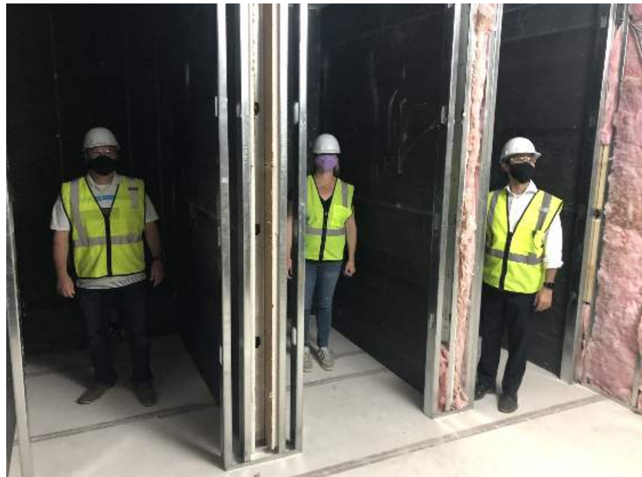
Inspecting the individual student restroom construction
