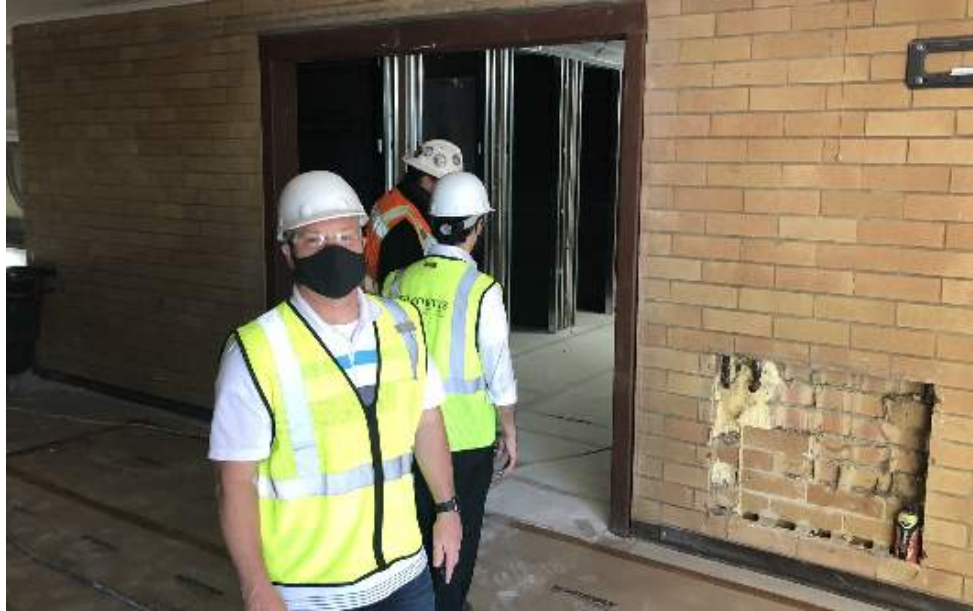
Superintendent Noss at the new individual student restroom entrance
