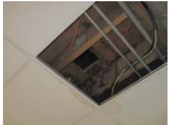
Figure A10.3.b – Roof joists
