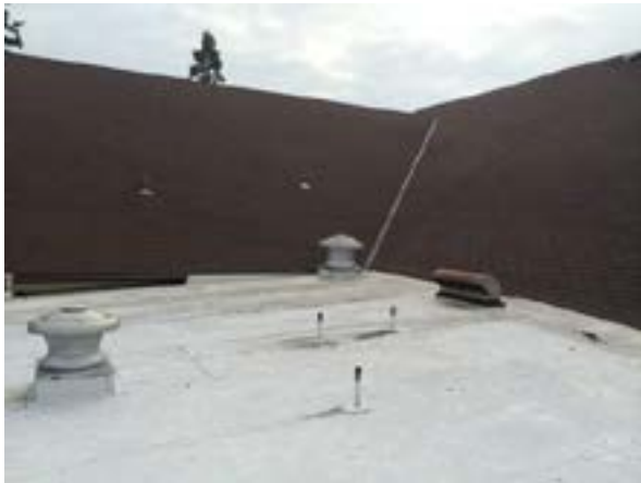
TPO Membrane is wearing out
