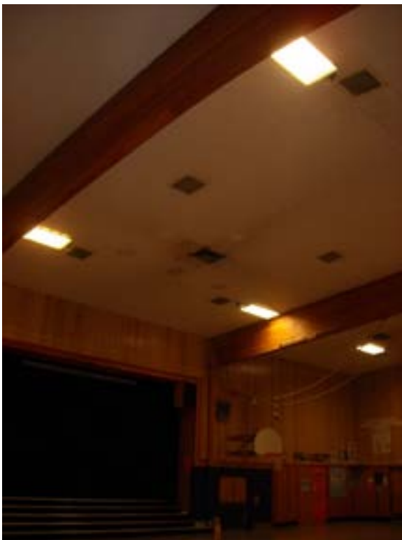
Figure B20.2 – Gymnasium ceiling
