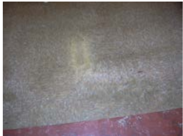
Figure B20.1 – Main office flooring
