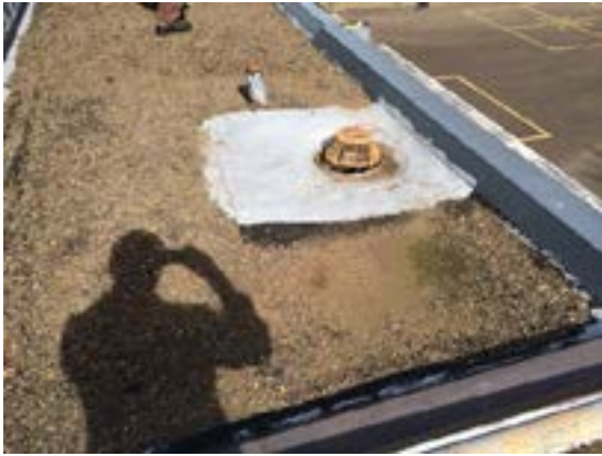
ROOF DRAINS HAVE BEEN PATCHED
