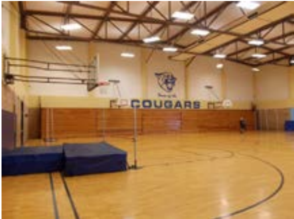
Figure B20.7 – Gymnasium bleachers
