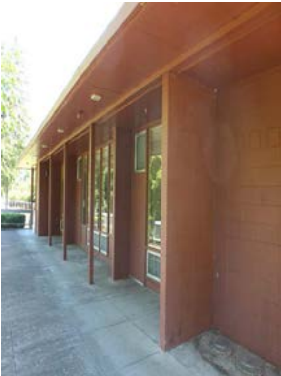
Figure E20.9.a – Incandescent lighting Figure
