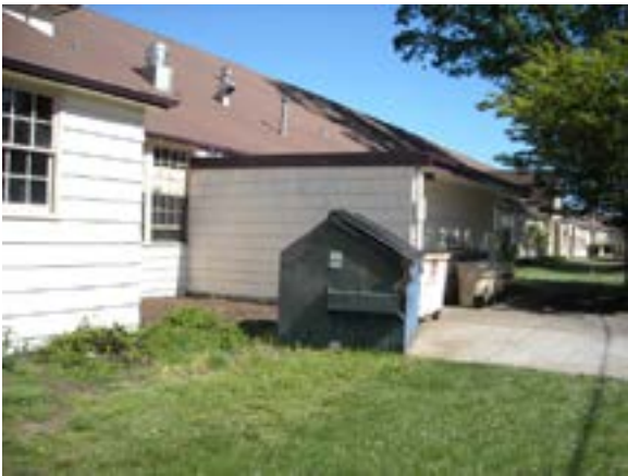
Figure E10.6 – Trash area
