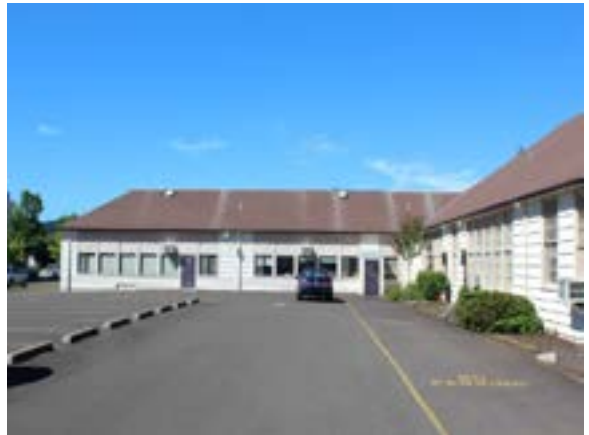
Figure E20.9 – Lack of parking lot lighting
