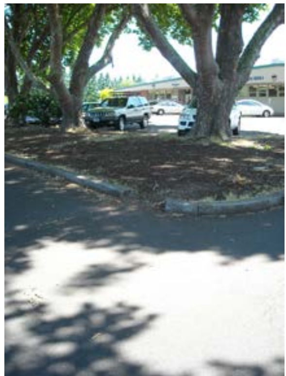
Figure E10.4 – Missing curb
