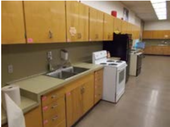
Figure B30.4 – Foods lab casework
