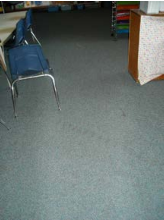
Figure B20.1.a – Carpeting in classroom
