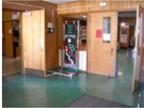
Figure B30.5 – Lack of visibility
