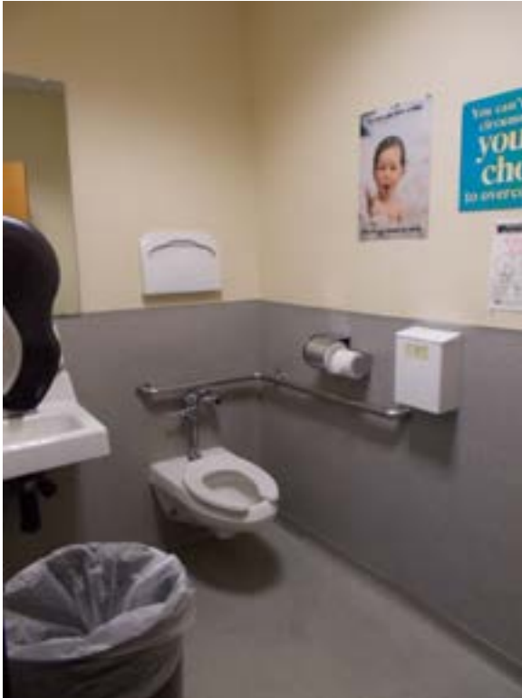
Figure B40.8 – Undersized toilet
