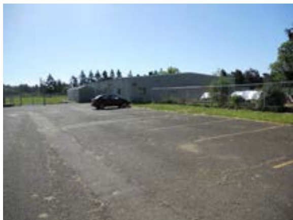
Figure E20.9.b – Perimeter lighting
