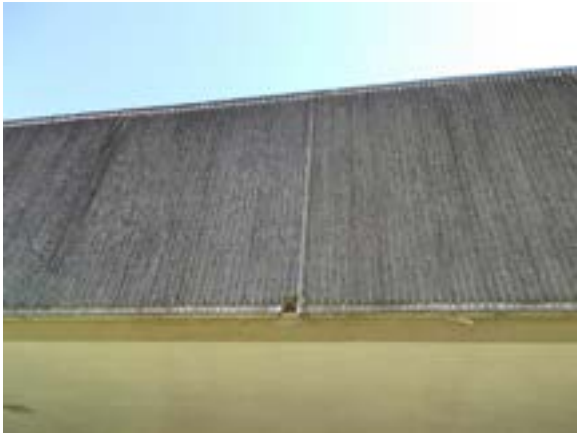
Figure A20.1 – Exterior Walls
