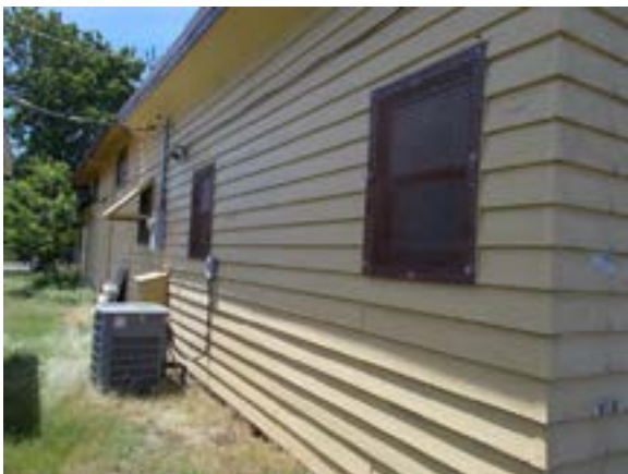
Figure A20.1 – Exterior walls
