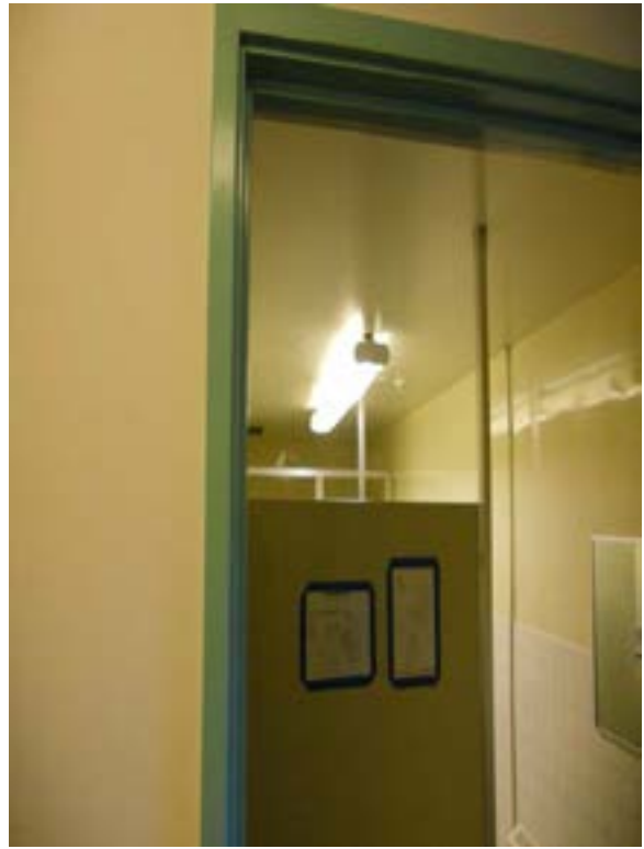
Figure D10.3.a – Light is missing lens
