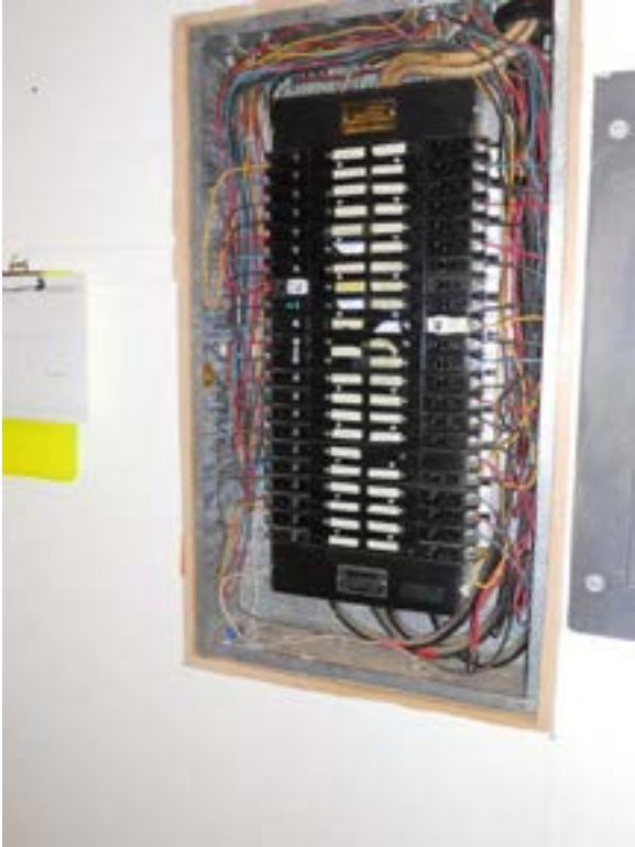
Figure D10.2.a - Typical panelboard
