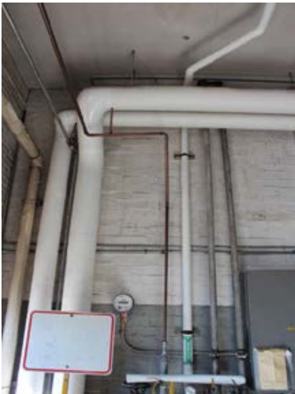
Figure D10.2.c – Piping installed above electrical
