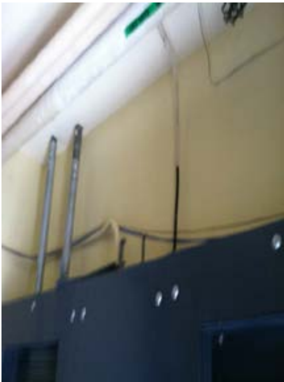
Figure D10.2.a - Pipes installed above panels
