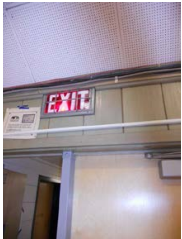
Figure D10.7 – Incandescent exit signs
