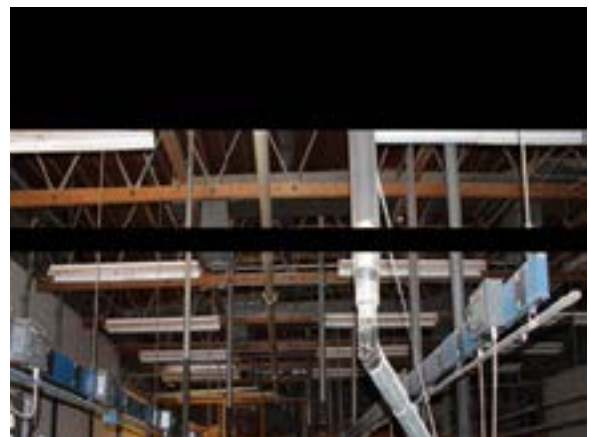
Figure D10.2.b – Aging busway system
