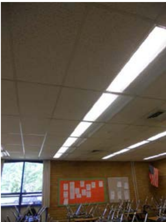
Figure D10.3 – Delamped classroom lighting
