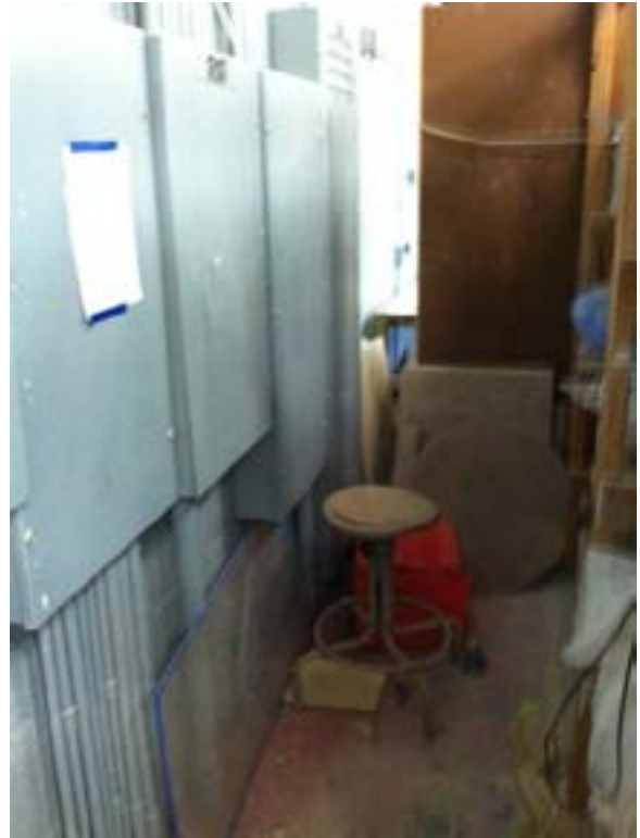
Figure D10.2.d – Electrical clearance
