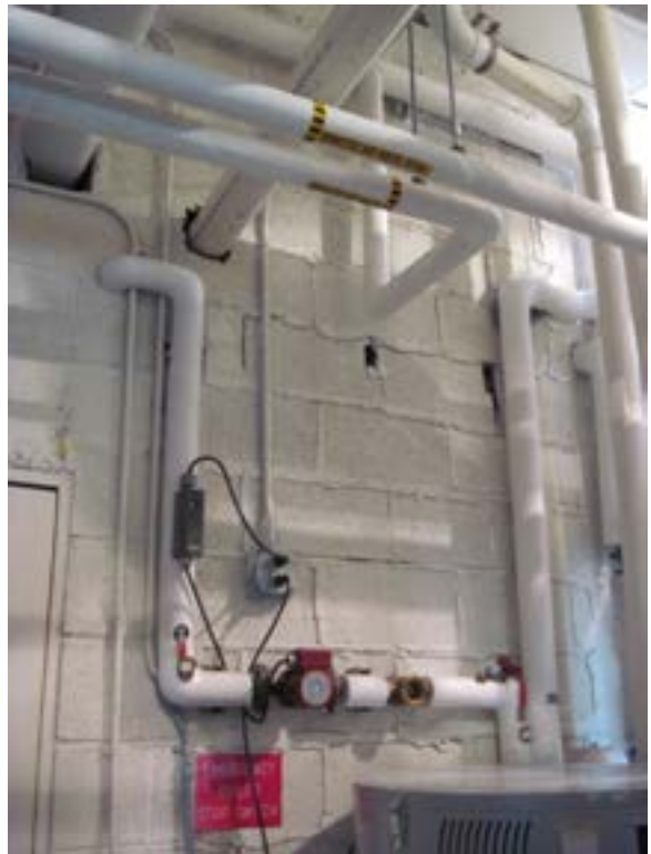
Figure A10.3.d – Boiler room wall
