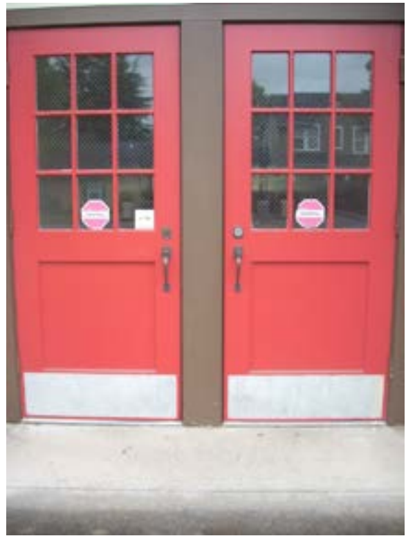
Figure A20.2.b – Gymnasium Doors
