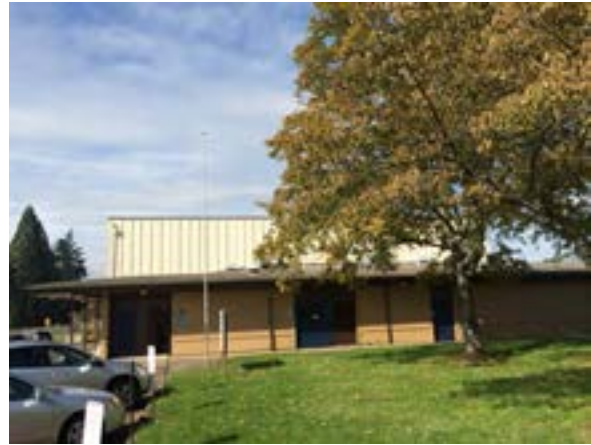
BUR NEARING END OF ITS USEFUL LIFE
