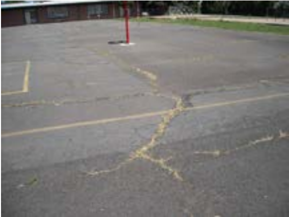
Figure E20.8 – Paving
