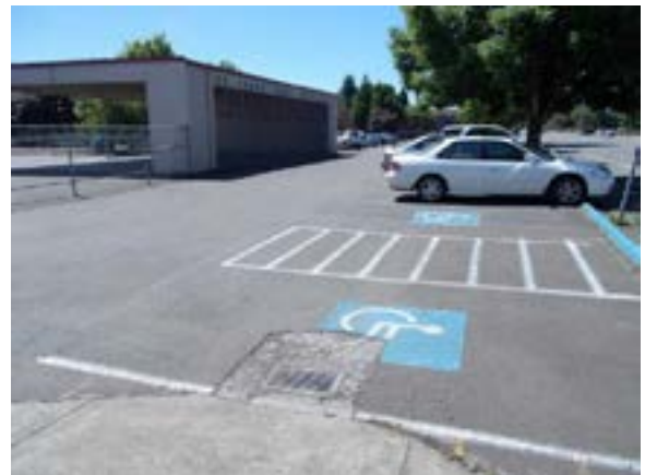
Figure E10.1.b – Parking lot
