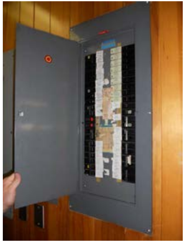
Figure D10.2.b - Multi-section branch panel
