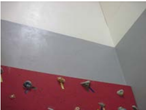
Figure A10.3.b – Cracks in panels
