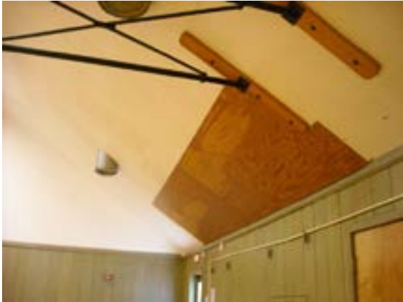
Figure B20.3 – Ceiling in gymnasium
