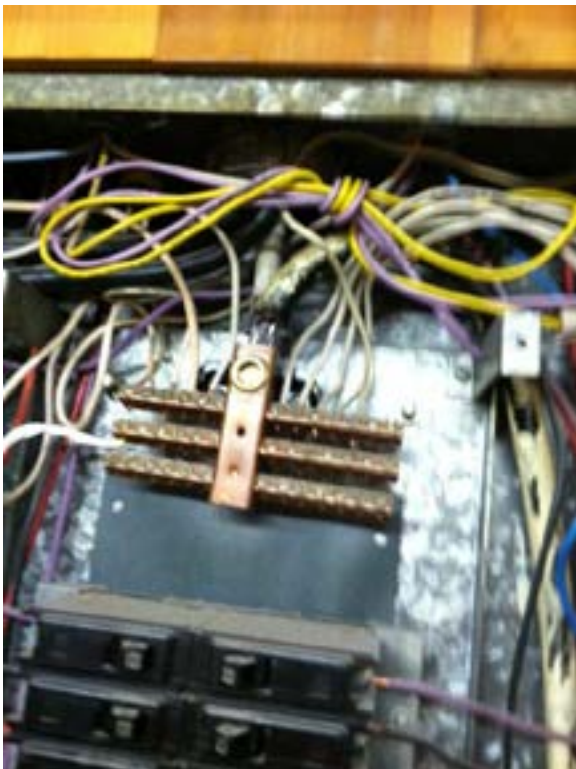
Figure D10.2.b – Neutral conductors share lug
