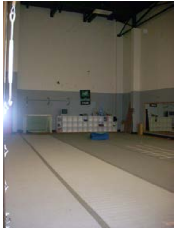
Figure B30.3 – Lack of acoustic treatment
