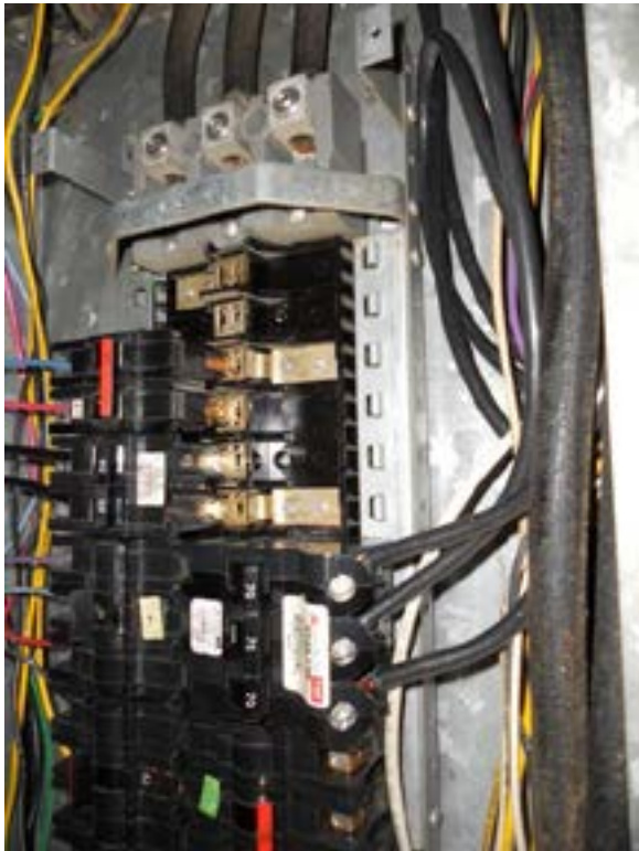
Figure D10.2.a – Typical panelboard
