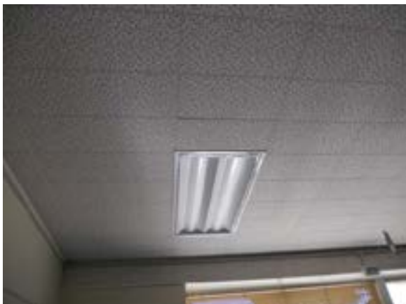
Figure D10.3.a – Classroom Light Retrofit
