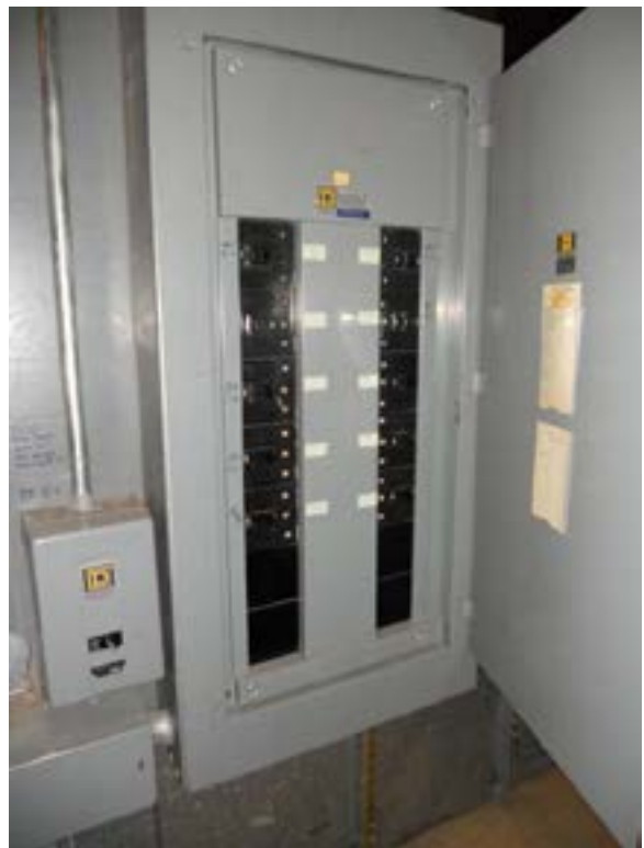
Figure D10.2.b – Typical panelboard
