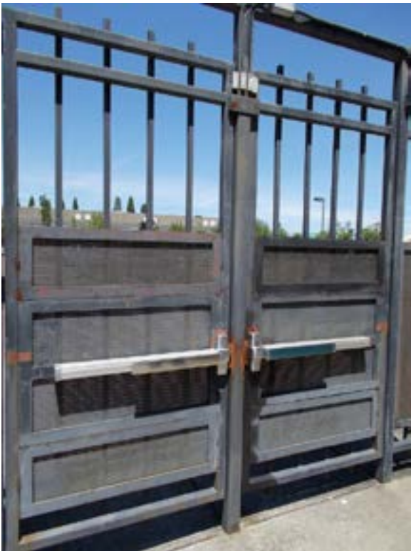
Figure E20.5 – Courtyard gate
