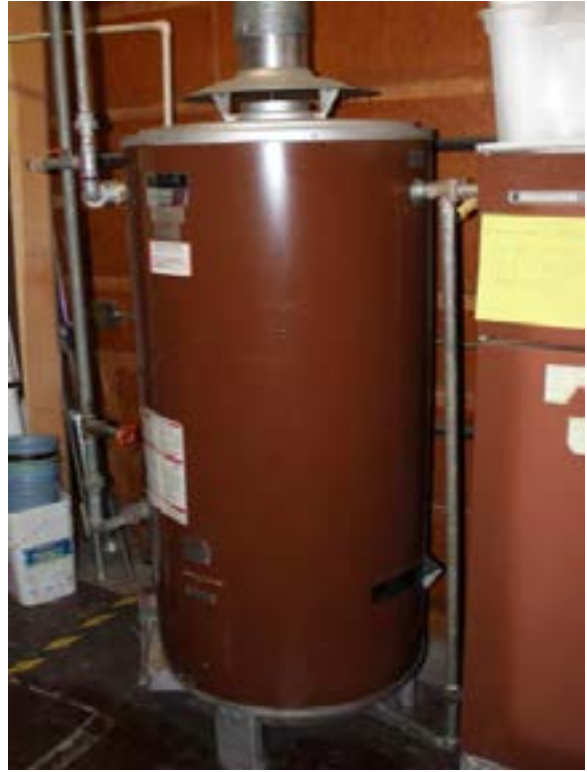
Figure C10.5 – Domestic hot water heater
