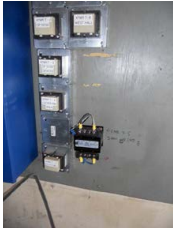
Figure D10.2.b – Control transformer
