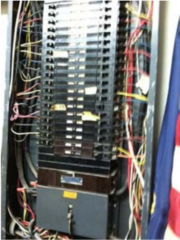
Figure D10.2.b – Panel missing grounding conductors and cover
