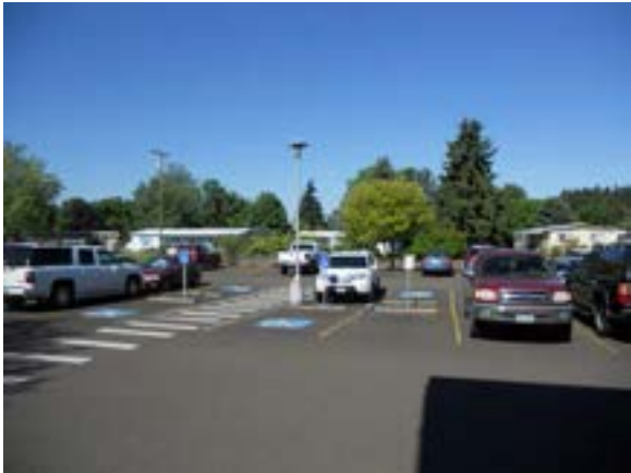
Figure E20.9 – Parking light poles
