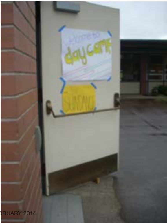
Figure A20.2 – Gymnasium door
