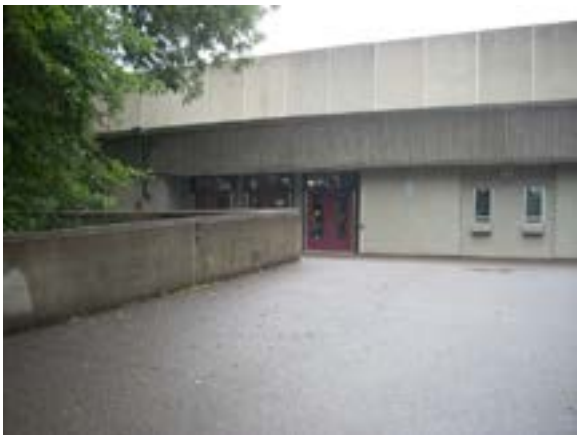
Figure B10.3 – Exterior ramp
