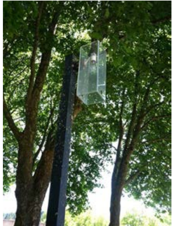
Figure E20.9.b - Unshielded lamps
