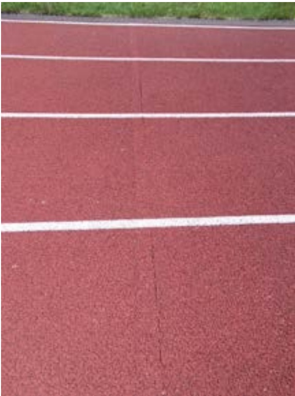
Figure E20.1 – Running track
