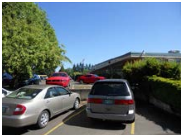
Figure E20.9.a – Administration building parking lot lighting
