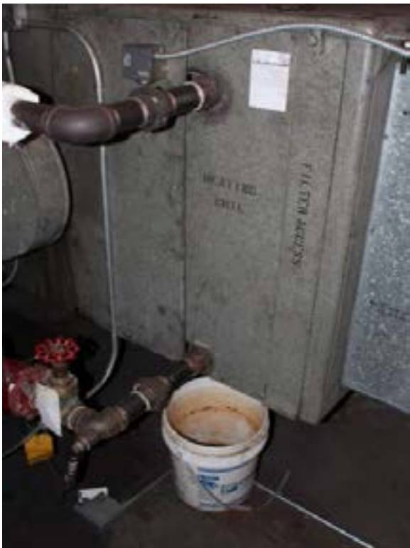
Figure C20.1 – Leaking coils
