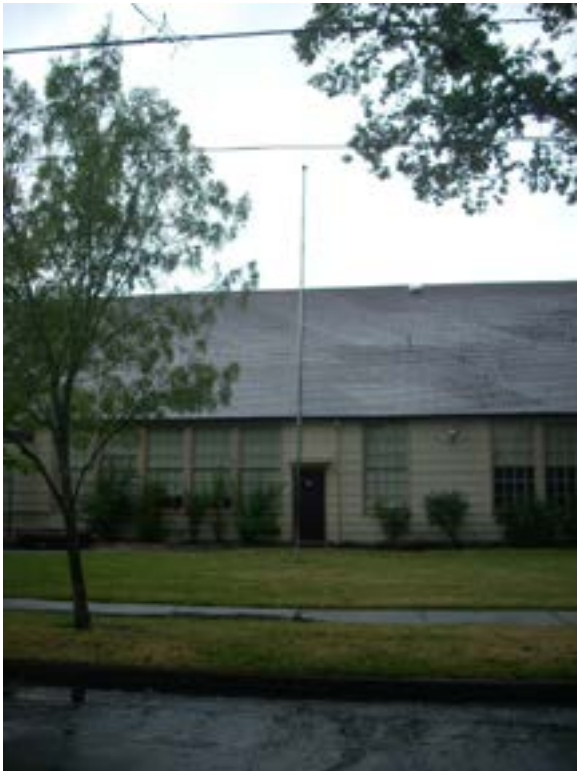
Figure E10.2 – Flagpole
