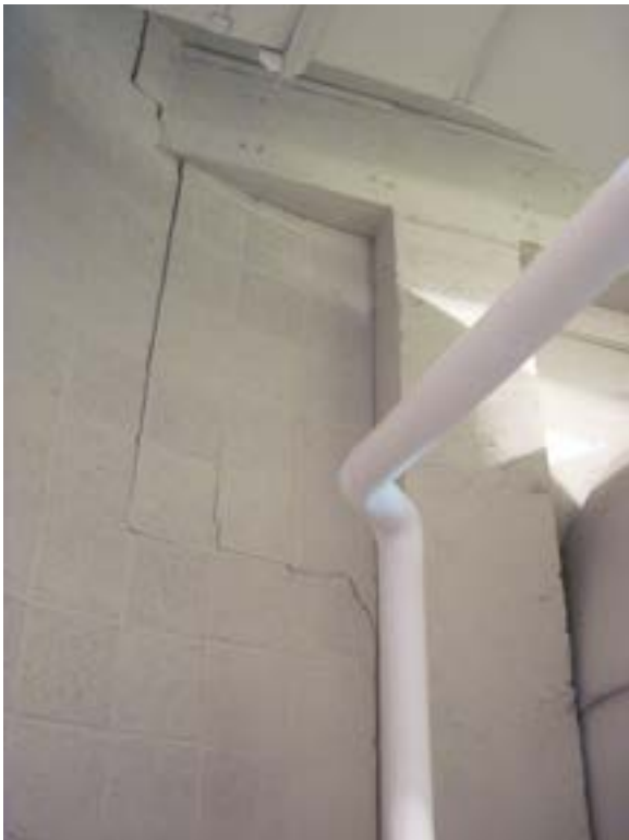
Figure A10.3.c – Boiler room wall
