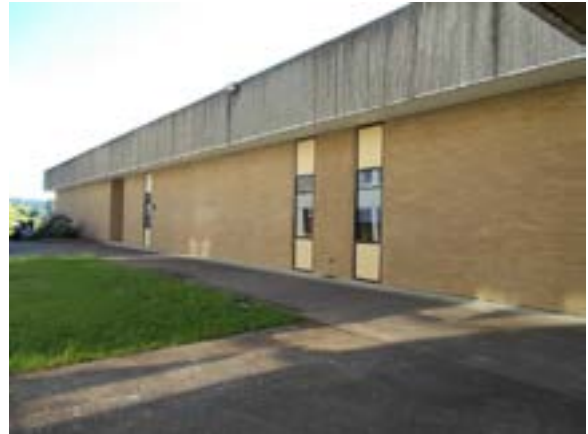
Figure A20.3.b – Exterior windows
