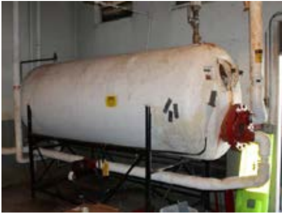
Figure C10.5 – Domestic hot water storage tank
