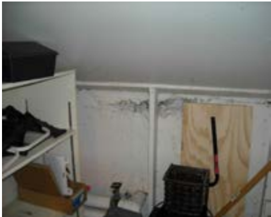
Figure A10.3 – Top of wall at lift
