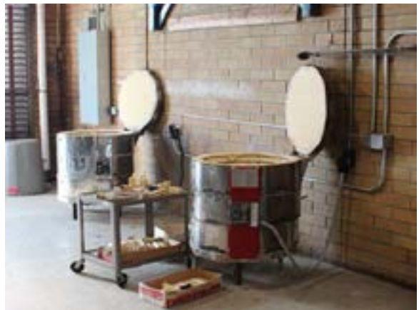
Figure C20.7 – Kilns in boiler room
