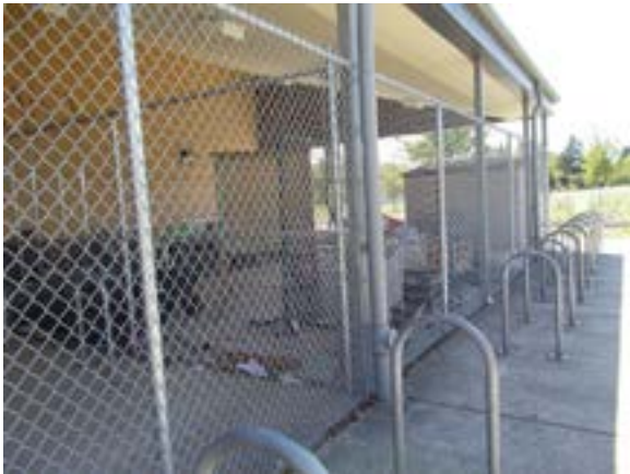
Figure E20.4 – Lack of site storage
