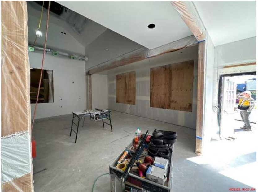
CHHS – New window openings at eating reception (view from inside)
