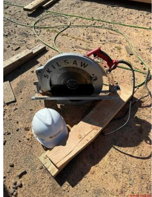
CHHS – One big saw (cutting large members)
