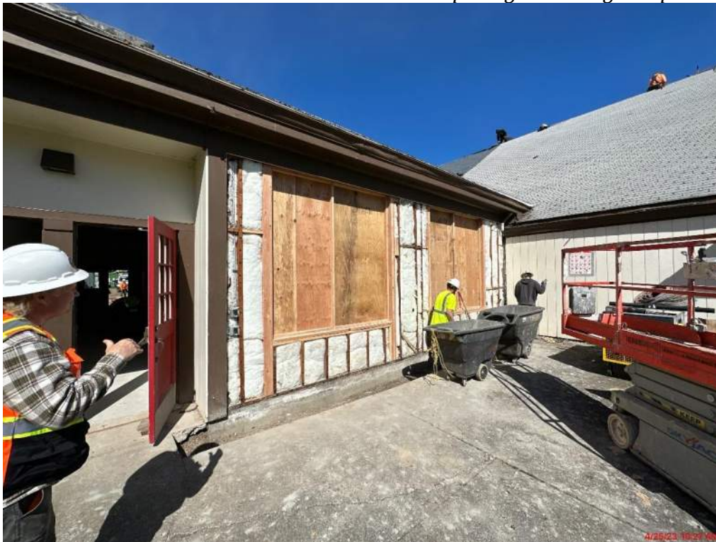
CHHS – New window openings (view from outside eating reception)
