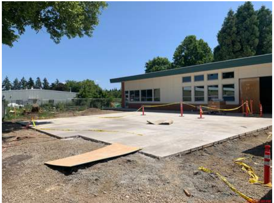
Exterior Hardscape Work
