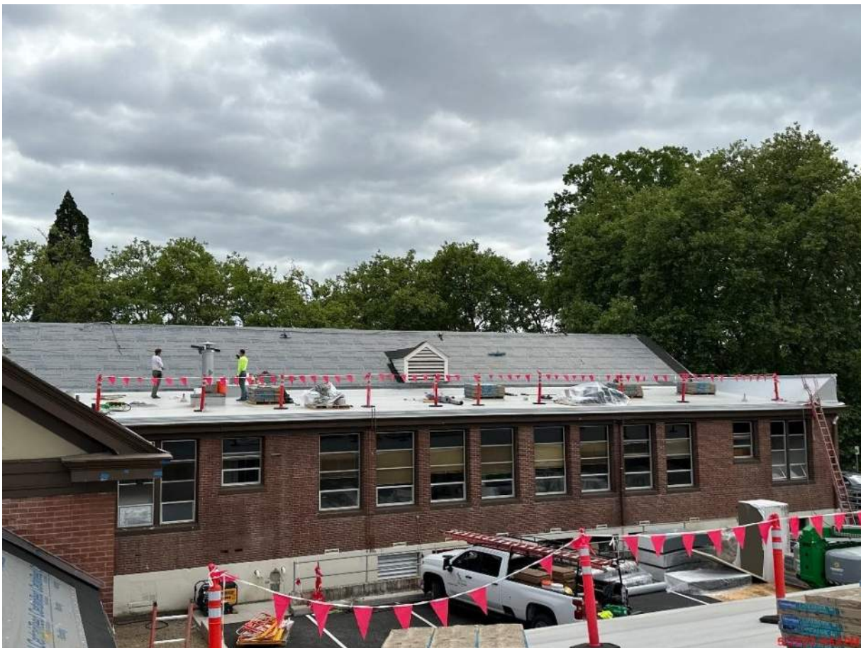
Harding Center / College Hill gets a new roof!
