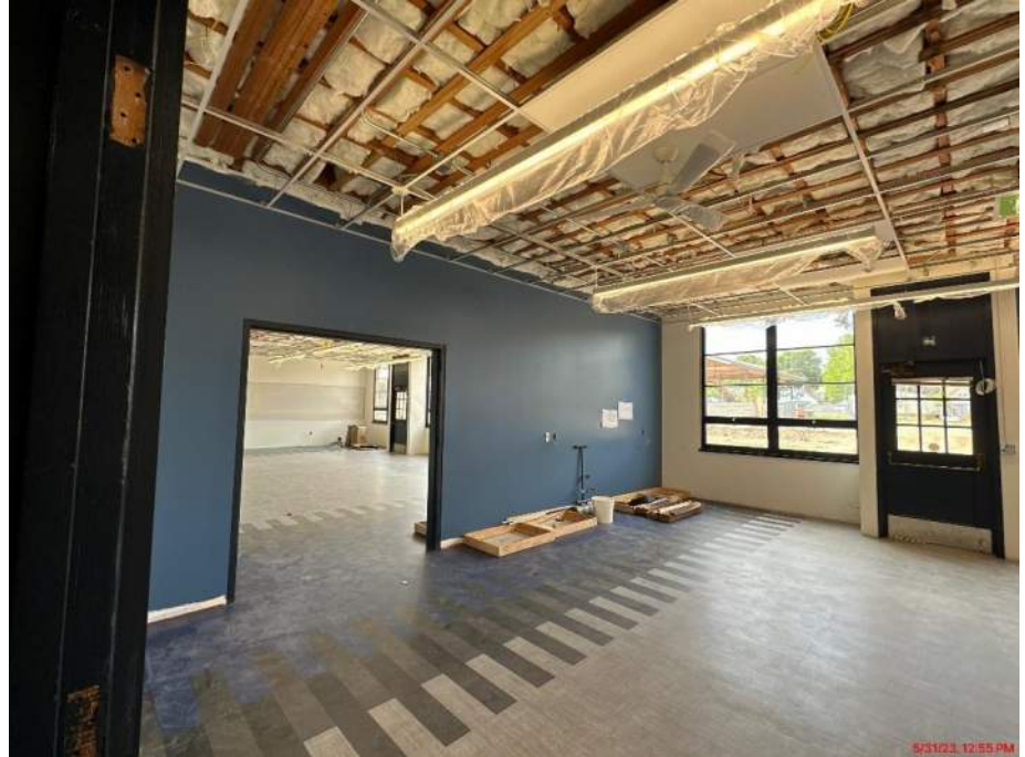
CHHS – Typical classroom finish progress (flooring, ceilings, lighting, paint)
