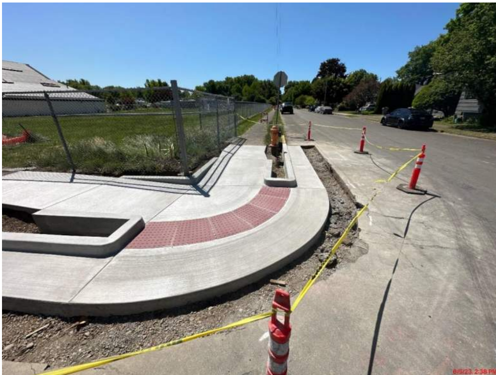
CHHS – New ADA PIPC work ready for pavement patching
