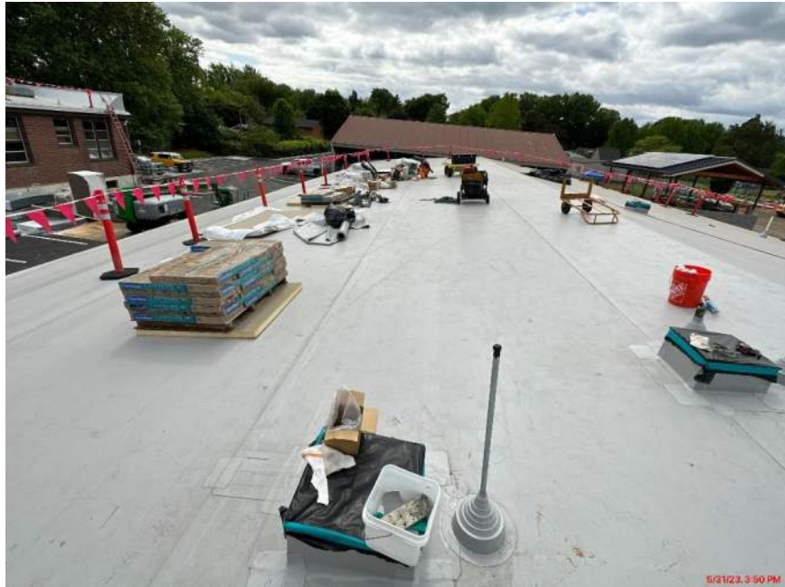
CHHS – Area B re-roof complete
