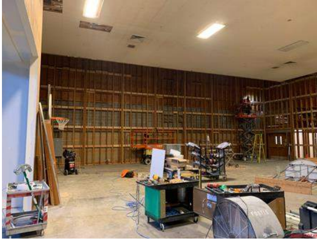
Gymnasium Seismic Work
