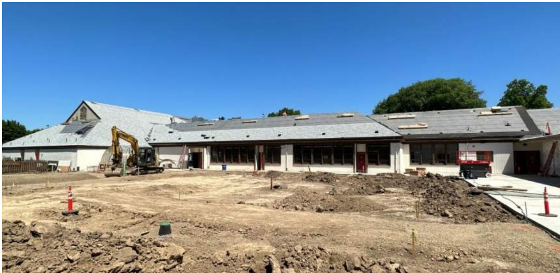
CHHS – New roof shingles and venting progress
