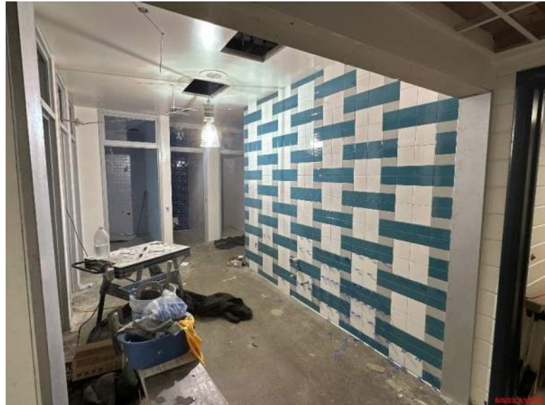
CHHS – Tile progress in restrooms throughout
