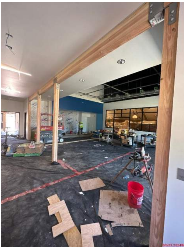
CHHS – Progress at reception eating area
