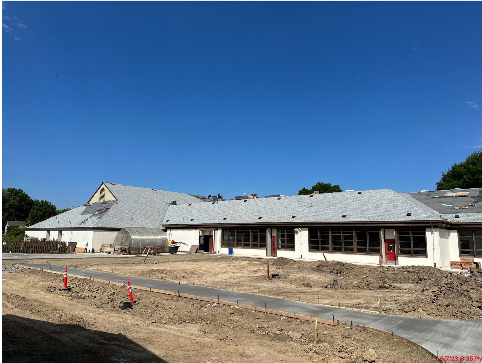
Roofing Progress and New Walkways
