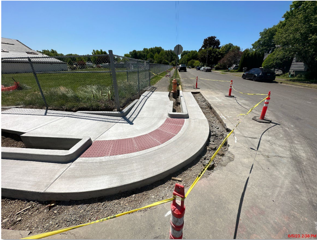
Exterior Improvements Underway
