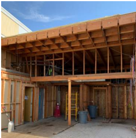
Former office area ready for new roof structure
