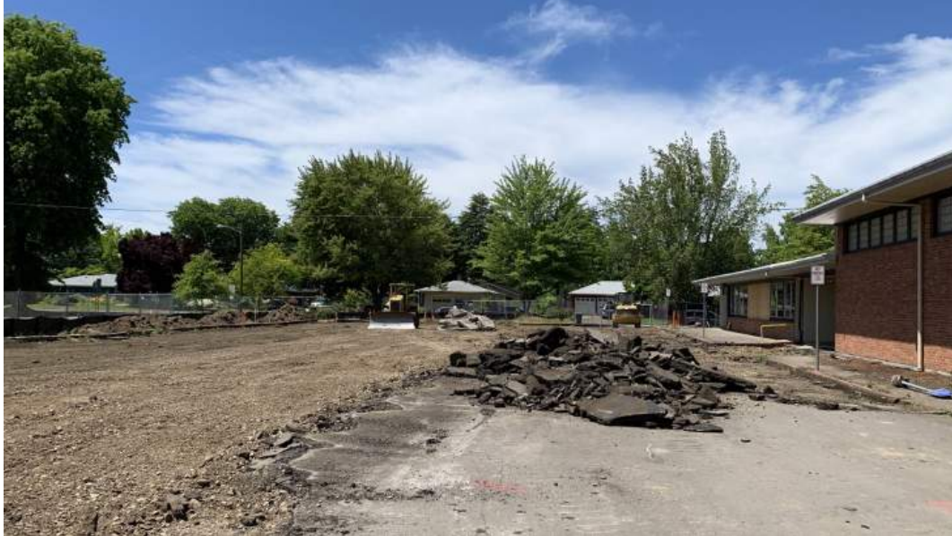
West parking lot under construction
