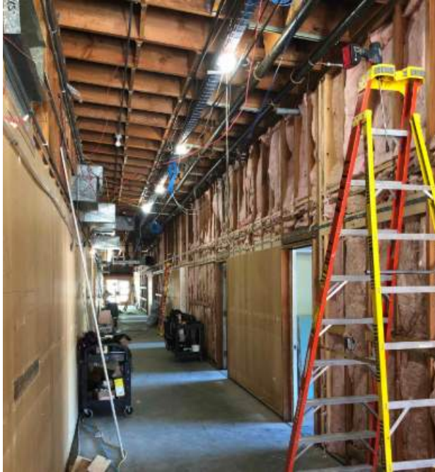
West corridor ceiling work, including seismic blocking, piping and electrical
